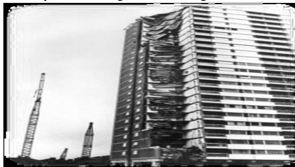
Fig. 1.1: Ronan point building after 1968
