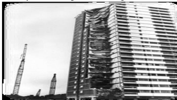
Fig. 1.1: Ronan point building after 1968
