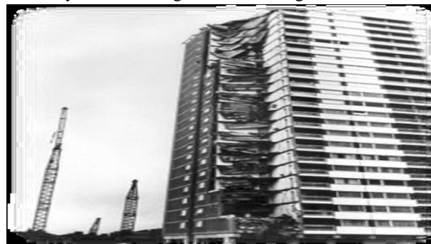
Fig. 1.1: Ronan point building after 1968
