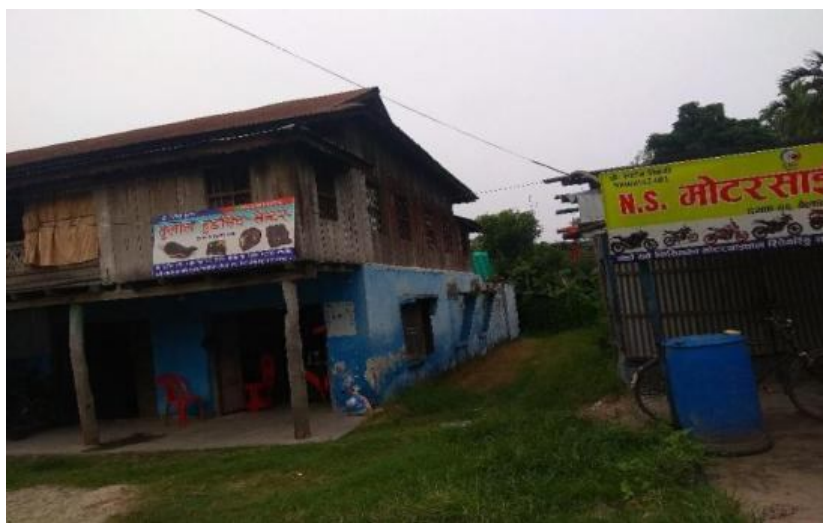
Fig. 12 Encroached public land
