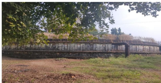
FIG 1. Water Tank (Panyacha Khajina)
