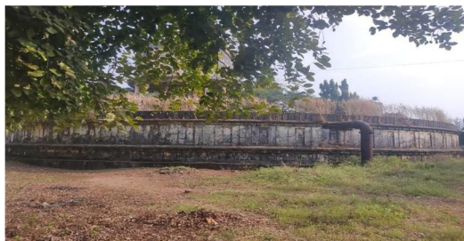
FIG 1. Water Tank (Panyacha Khajina)
