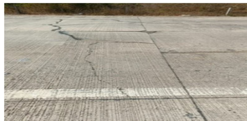
Transverse Cracks
