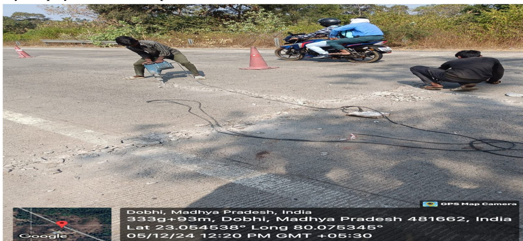
Fig.4 Filling of joints using bitumen sealant
