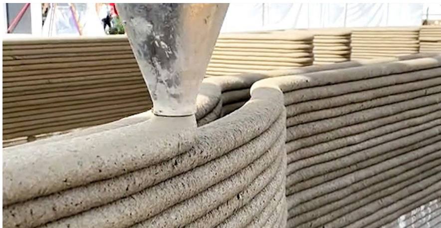
Figure 1. 3DCP in Processing
