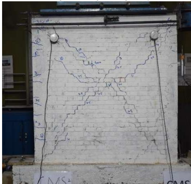
Figure 7: Damage pattern before retrofitting
