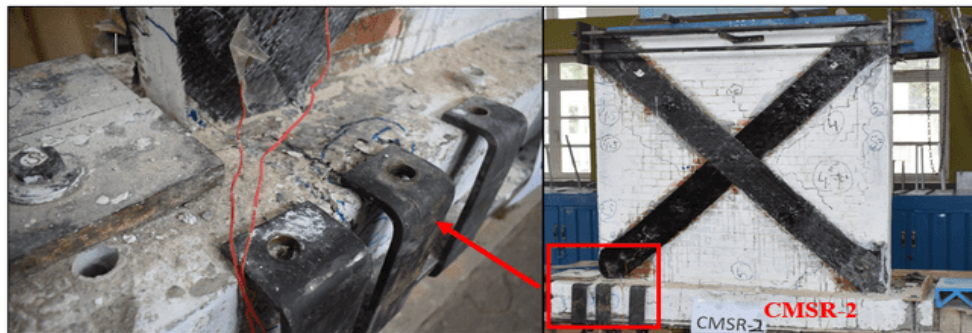
Figure 10. Crack pattern and failure mode after Retrofitting
