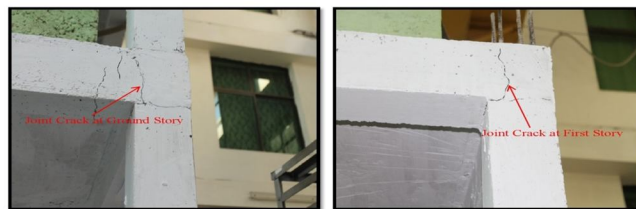
Beam-Column Joint Crack at Ground Story
