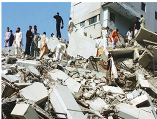
Figure 1.1: Collapse of Reinforced Concrete Structure in past earthquakes
