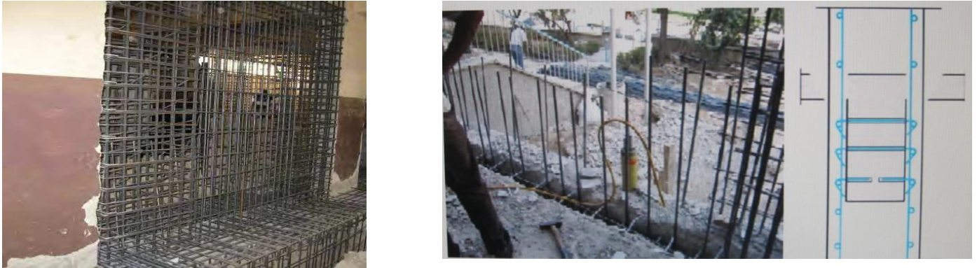
Fig. 2 System based strengthening of RC members
