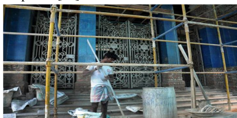
Fig4. Wrapping the Chennai Corporation Building with Fibre
