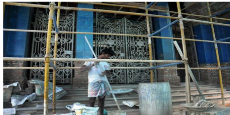
Fig4. Wrapping the Chennai Corporation Building with Fibre
