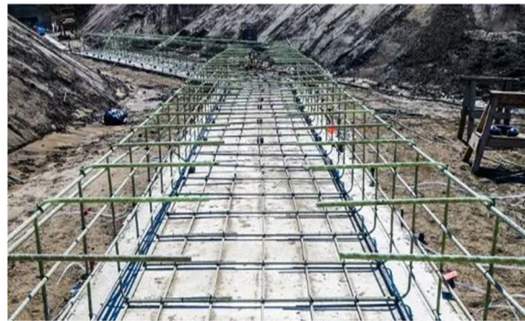
CFRP bars are used in reinforced concrete structures
