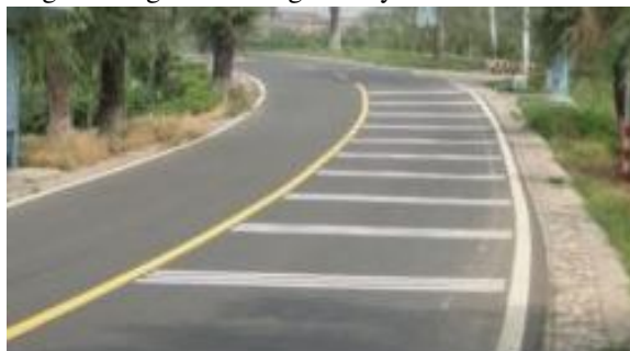
Fig.7 Optical marking on curve.
