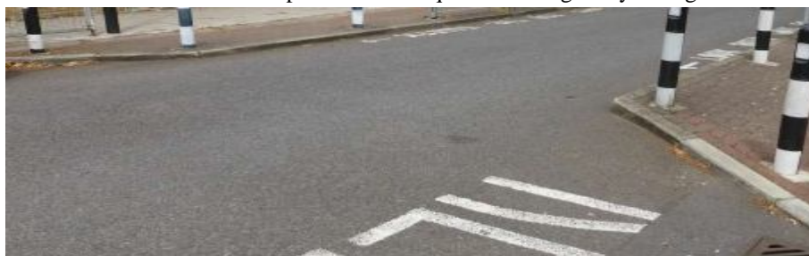
Fig.5 Road narrowing near a school in the UK
