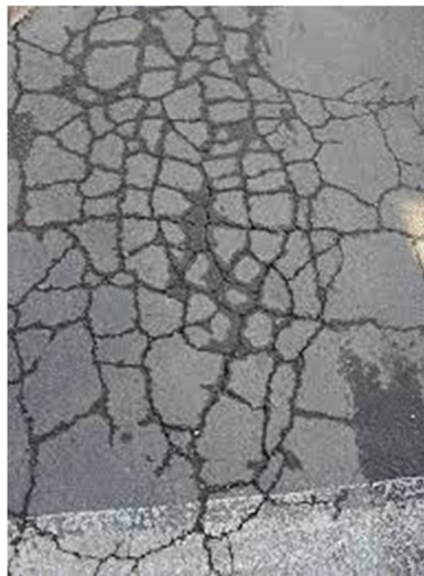
Figure 2: Alligator cracks.
