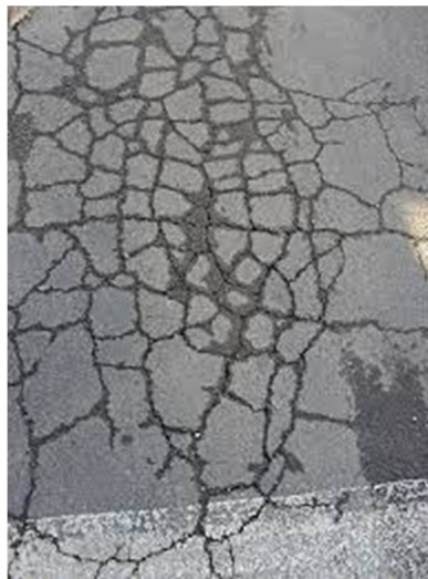
Figure 2: Alligator cracks.
