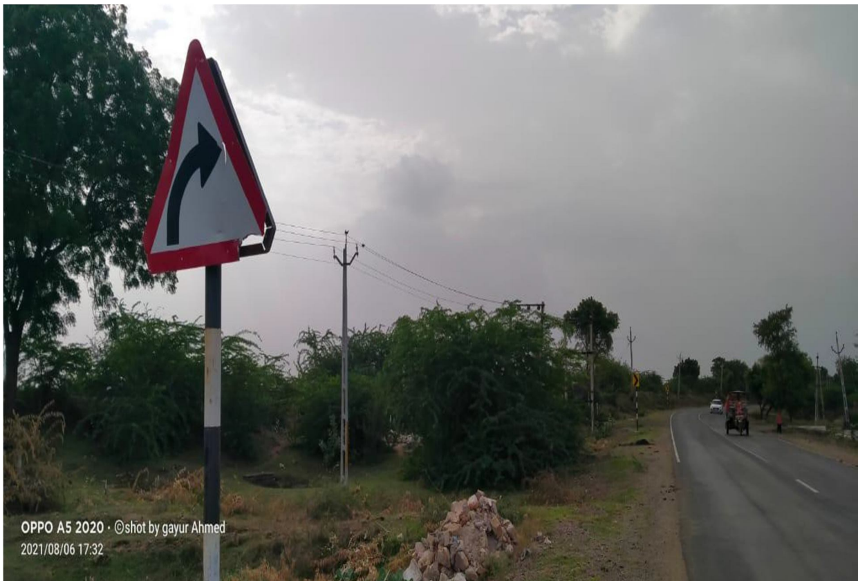
Ch. 3+635 Left turn sign board found in damaged condition & construction material dumped near shoulder
