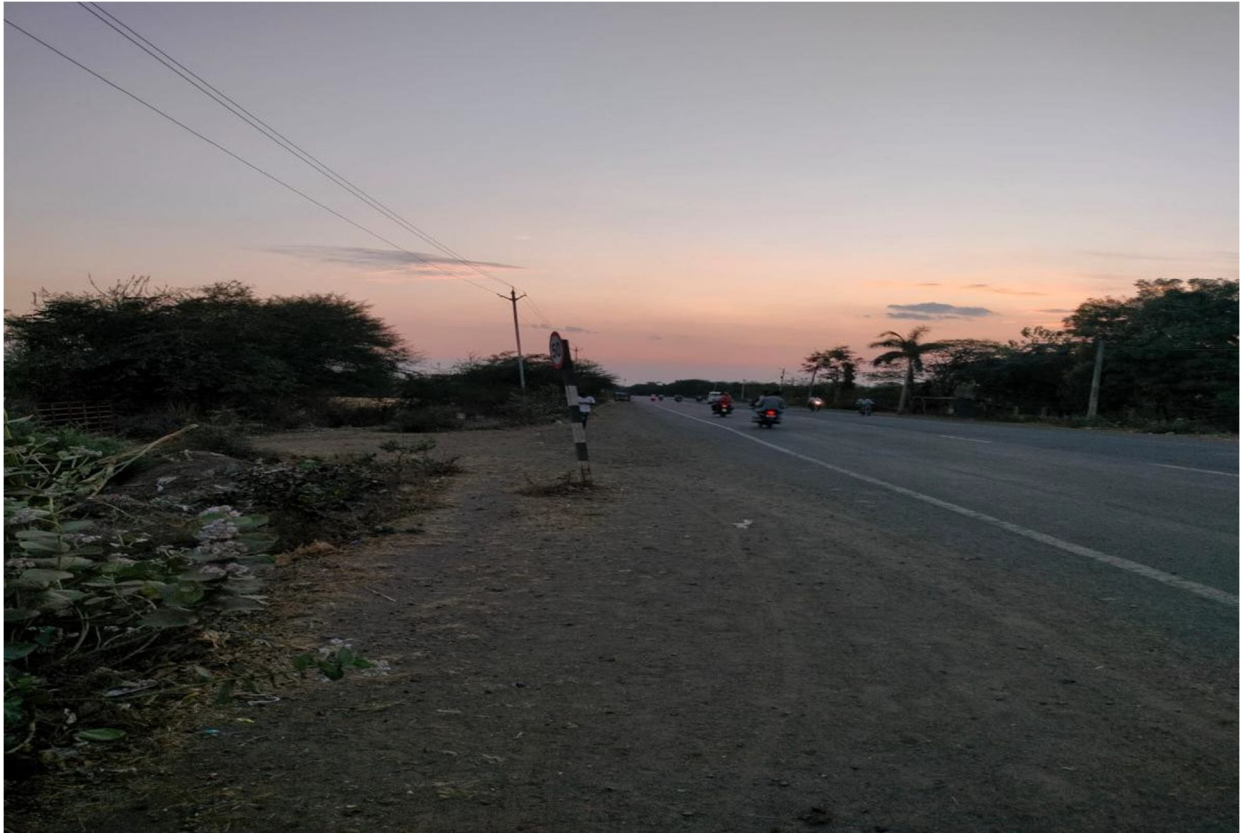
Ch. 20+560 Damaged Speed Limit Sign Must be repaired
