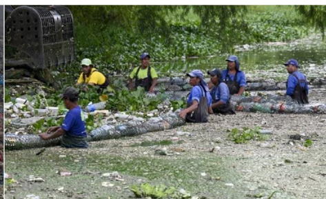
Fig.2: cleaning water surfaces manually
