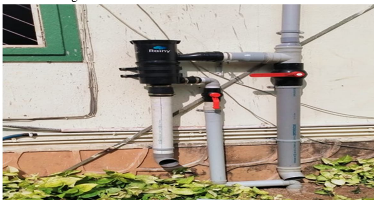
Fig. 2 Components of rooftop rainwater harvesting
