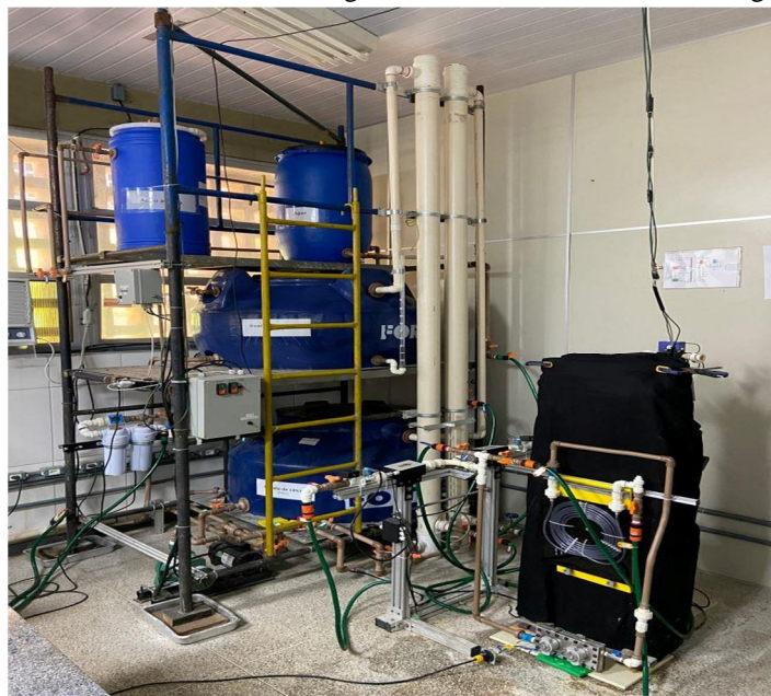
Fig. 2 Image of the calcium carbonate scaling plant.
