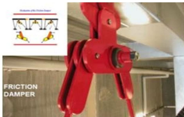
Fig1: Friction Damper
