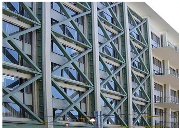
Fig. Infill shear trusses
