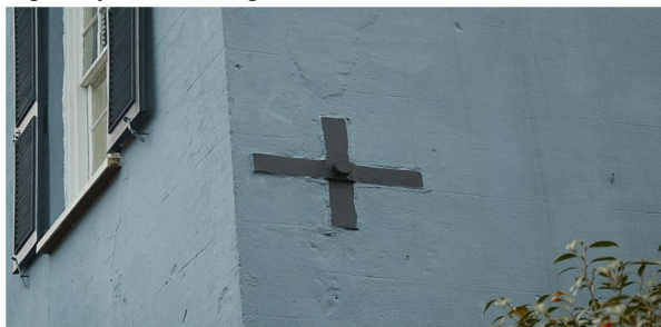
Fig. External post-tensioning
