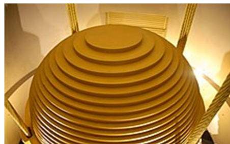
Fig. Tuned mass dampers
