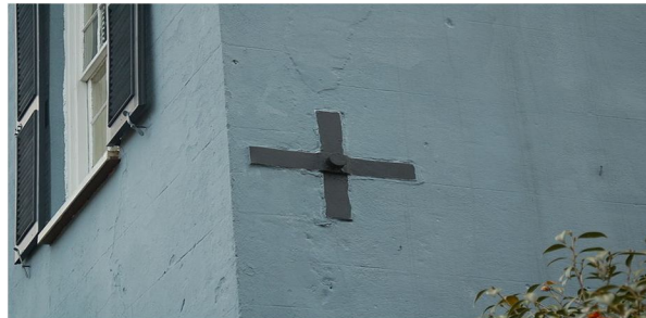
Fig. External post-tensioning
