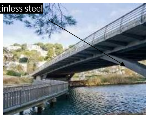
Fig. 1.2 Cala Galdana Bridge ( www.worldstainless.org )
