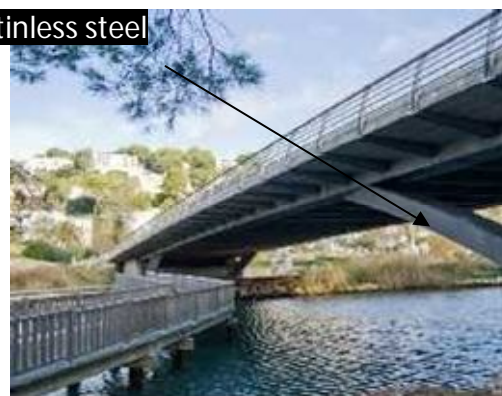
Fig. 1.2 Cala Galdana Bridge ( www.worldstainless.org )
