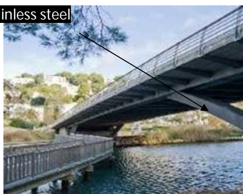
Fig. 1.2 Cala Galdana Bridge ( www.worldstainless.org )
