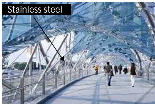
Fig. 1.3 Helix Pedestrian bridge ( www.e- architect.co.uk )
