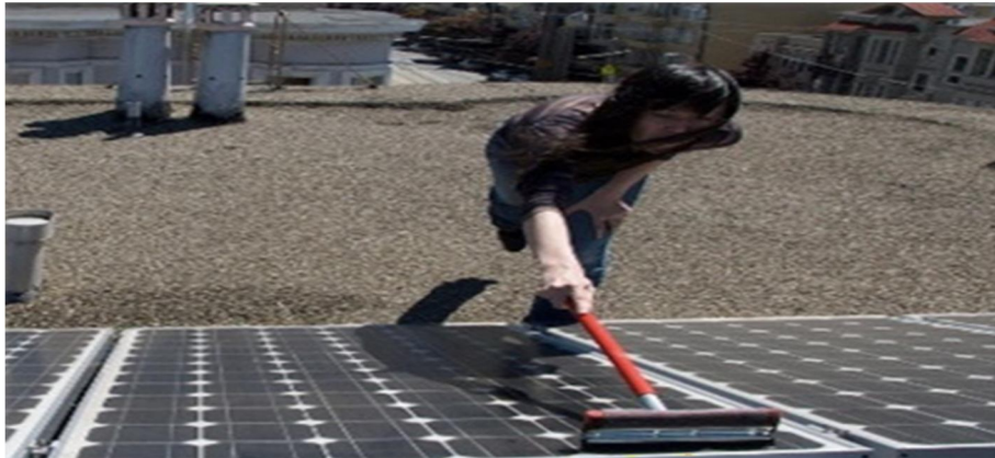
Figure 2 Manual cleaning of Solar Panel
