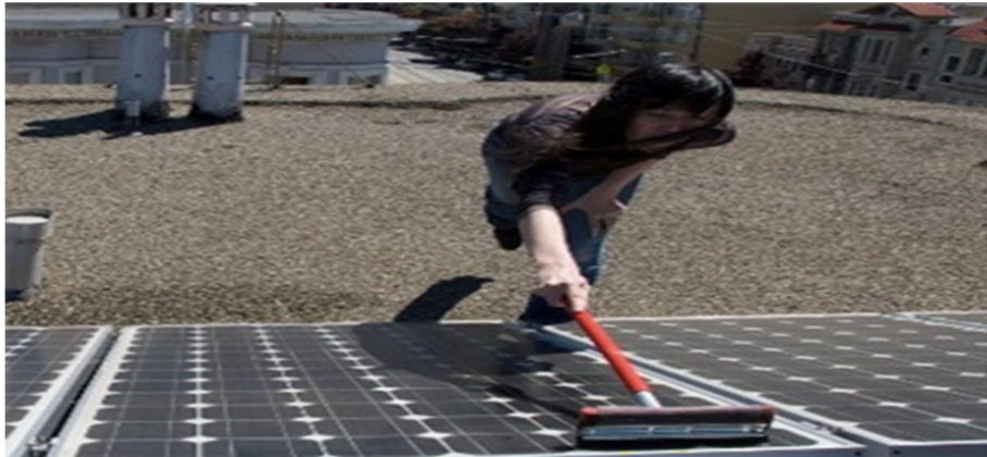
Figure 2 Manual cleaning of Solar Panel
