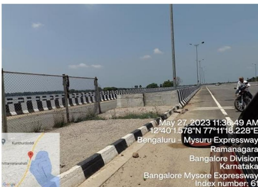
No Advance Warning About Curve/Cheron Marker/Delinator
