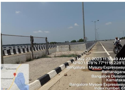
No Advance Warning About Curve/Cheron Marker/Delinator
