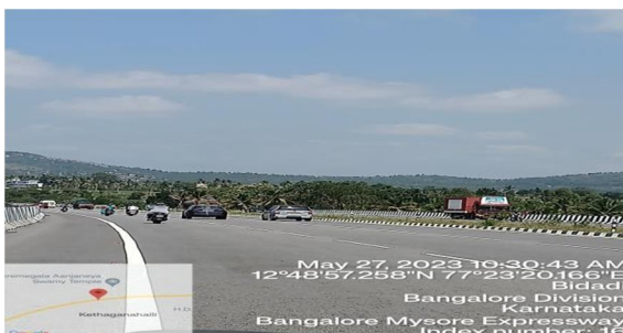
No Advance Warning About Curve/Cheron Marker/Delinator
