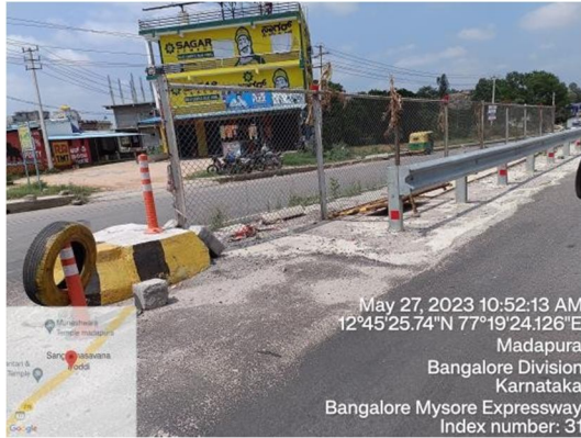
No Dip Sign Board/No Advance Warning
