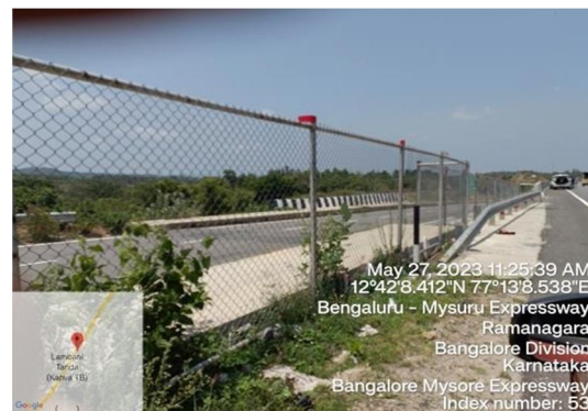
No Advance Warning About Curve/Cheron Marker/Delinator
