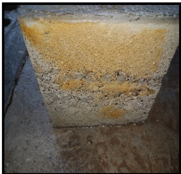
Photo 1- Cube showing effect of acid after immersion in H2SO4 solution
