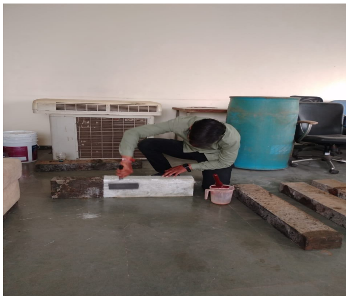
Figure 1. Application of GFRP
