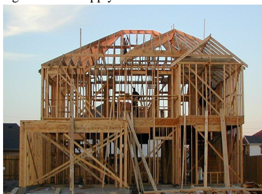
Fig 3. A Wood – Framed House Under Construction in Texas, United States
