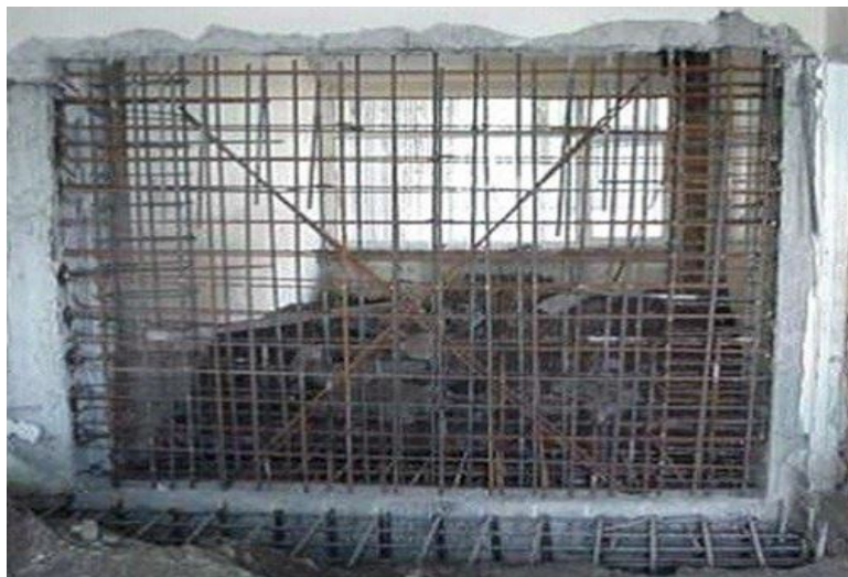
Fig1.1 Additional Shear Wall
