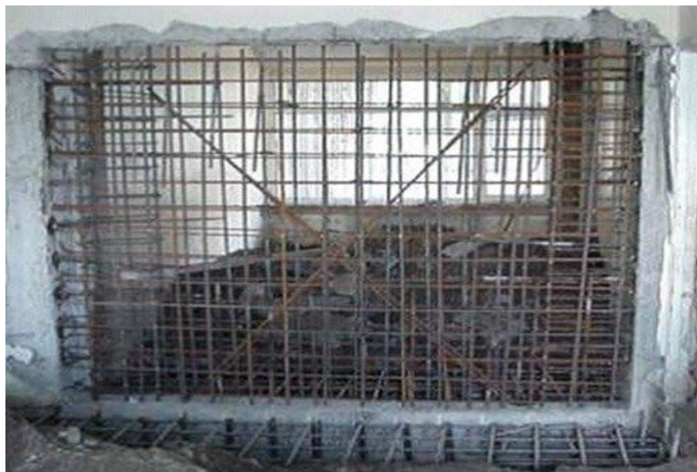
Fig1.1 Additional Shear Wall
