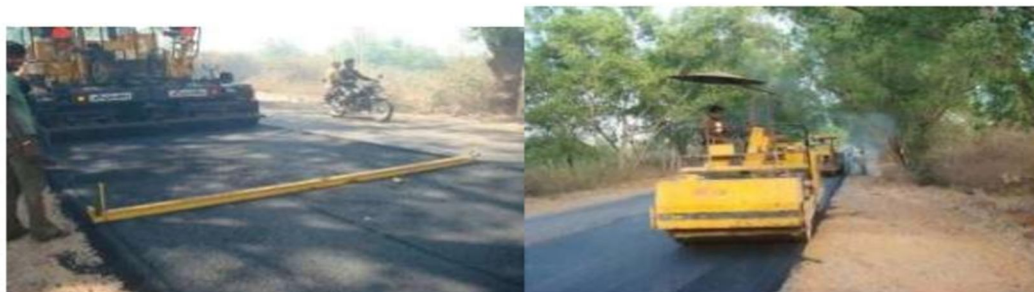
Figure 34 Overlay construction: Compaction
