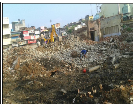
Fig 2 : Demolished aggregates on site
