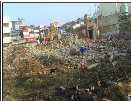
Fig 2 : Demolished aggregates on site
