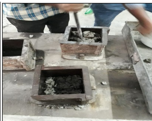
Fig 5: Preparation of Cubes
