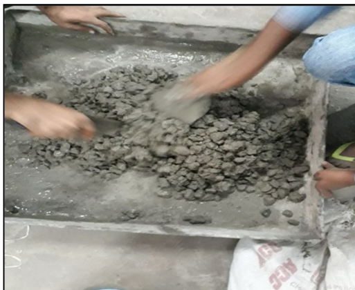
Fig 4: Mixing of Aggregates
