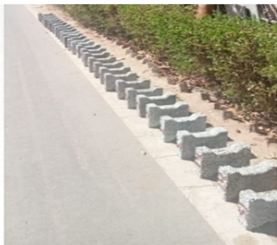
Image D ppb drying in sun light
