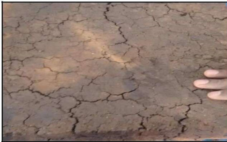
FIG 5.1: BC Soil Shrinkage Cracks after testing
