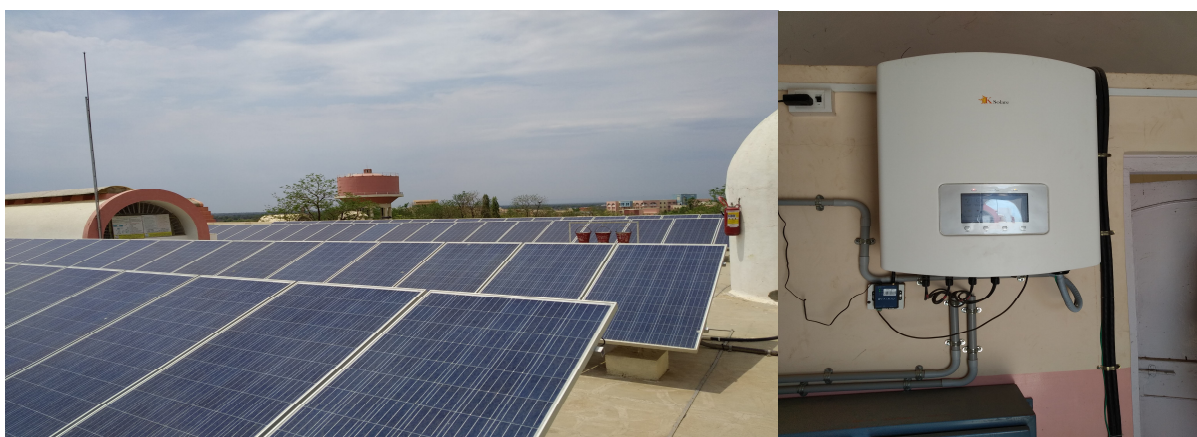
Fig.6 Grid Connected Roof-Top(GCRT) Solar PV system
