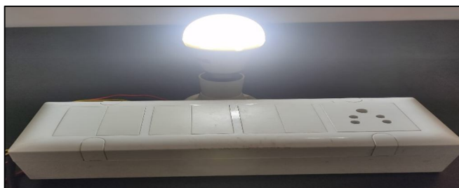
Figure 8 : Working view of project
