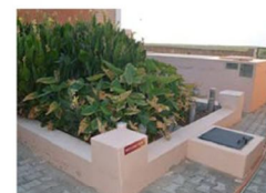
Energy efficient and eco-friendly phyto-remediation STP plant
