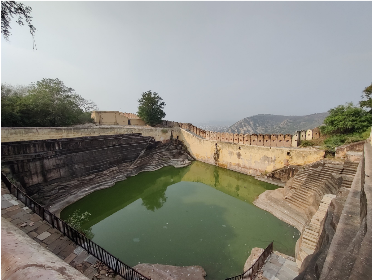
Figure 7: Rain water collecting tanks on fort complex
