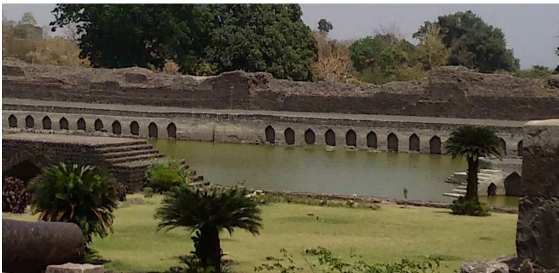
Figure 10: Embankments of Kapoor talab
