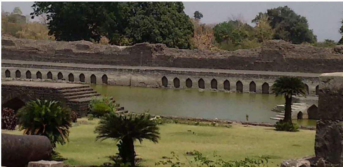
Figure 10: Embankments of Kapoor talab
