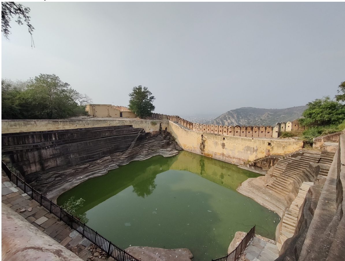
Figure 7: Rain water collecting tanks on fort complex
