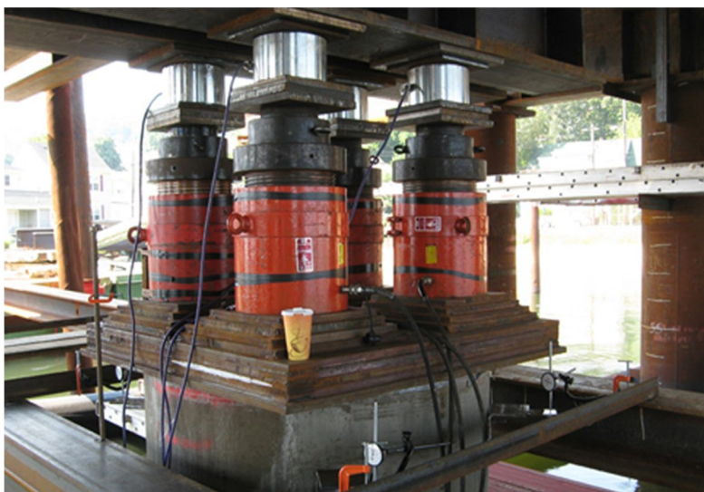
Figure No. 3 Demonstration of hydraulic jack in footpath
