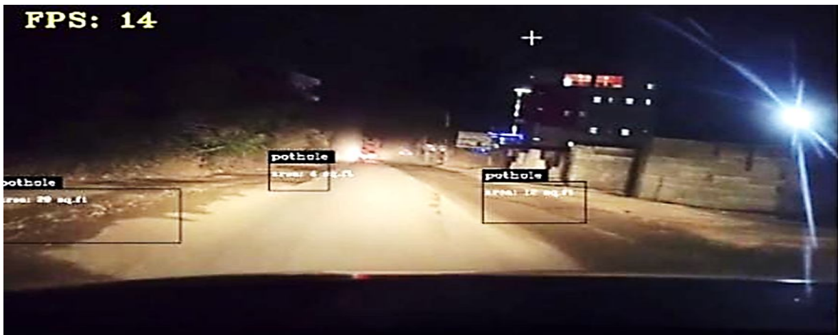
Figure 5: Detection of pothole during night
