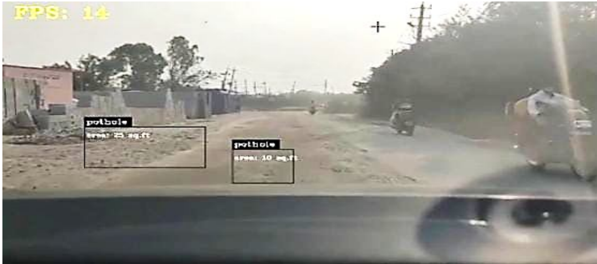
Figure 4 : Detection of pothole during day
