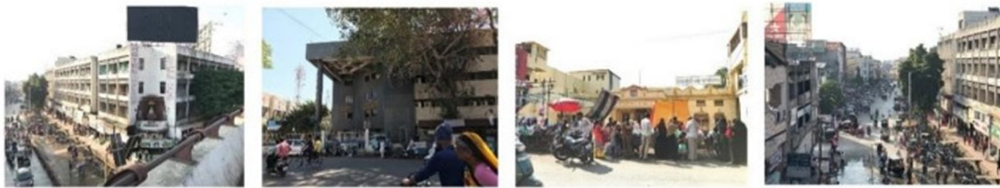
Administrative Buildings (AMC, BSNL office, City Library and Market area).
