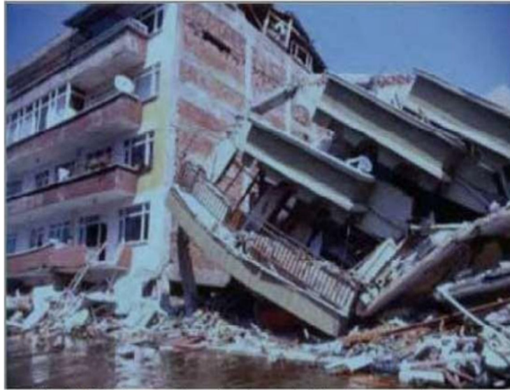
Fig. 1. Multiple-story collapse in a six-story building due to strong beam-weak column design in the 1999 Turkey earthquake.
