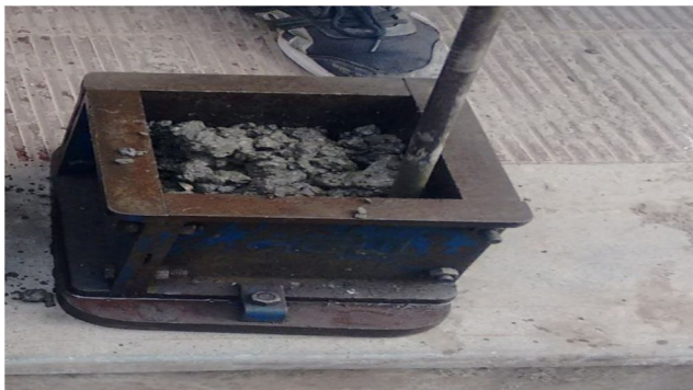
Fig 4.7 Placing of concrete in moulds
