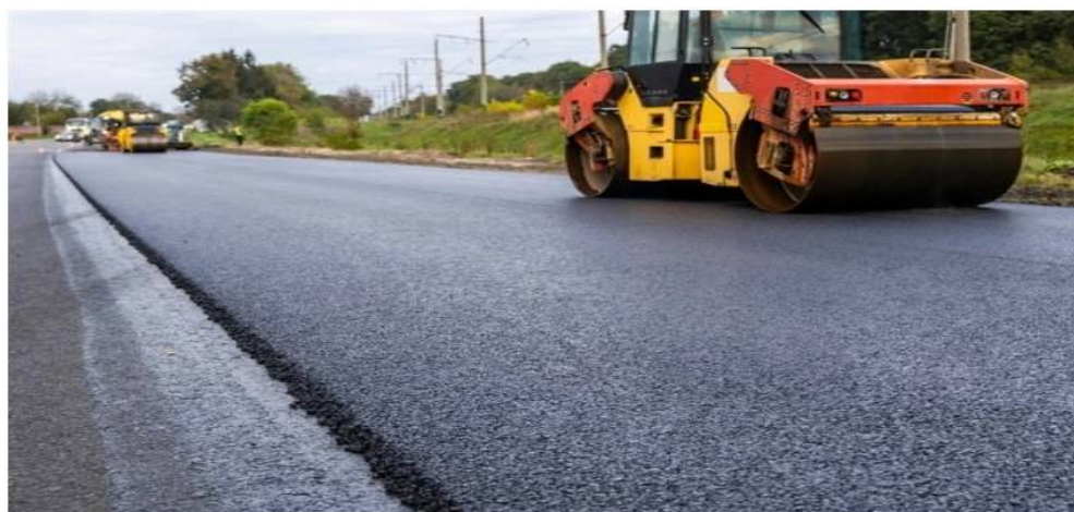
Figure:- 5.1(a) Paving Road using waste tyres.
