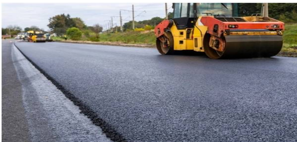
Figure:- 5.1(a) Paving Road using waste tyres.
