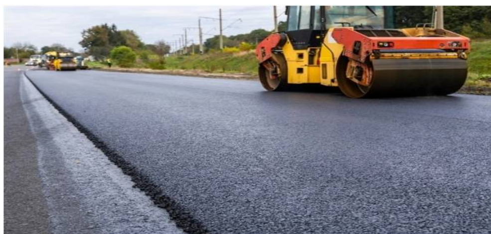
Figure:- 5.1(a) Paving Road using waste tyres.
