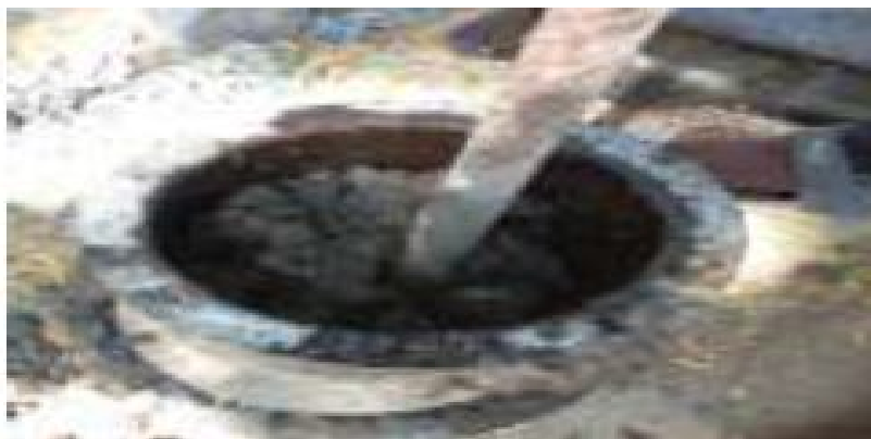
Fig 3.3 :-Casting of cylinders
