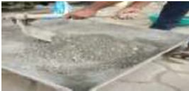
Fig 3.1 :-Mixing of materials
