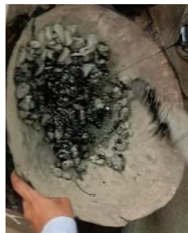
Fig-4: Mixing of Bitumen
