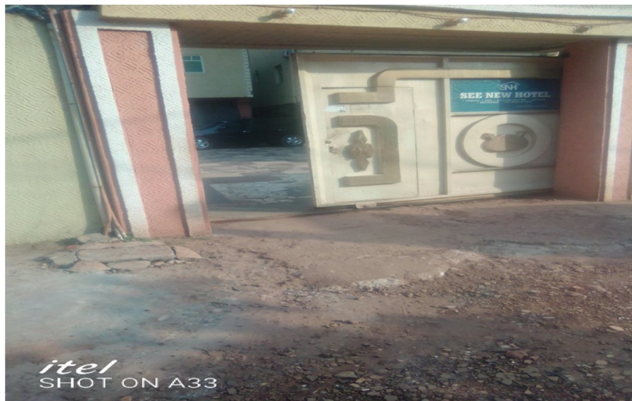
Figure 5.1 shows an entrance of an existing hotel in Nsukka Source: (Filed Survey).
