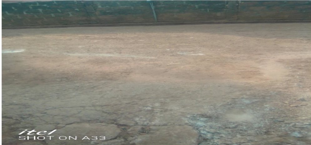
Figure 5.4 shows the state of dilapidated floor finishes leading to a hotel in Nsukka Source: (Filed Survey).
