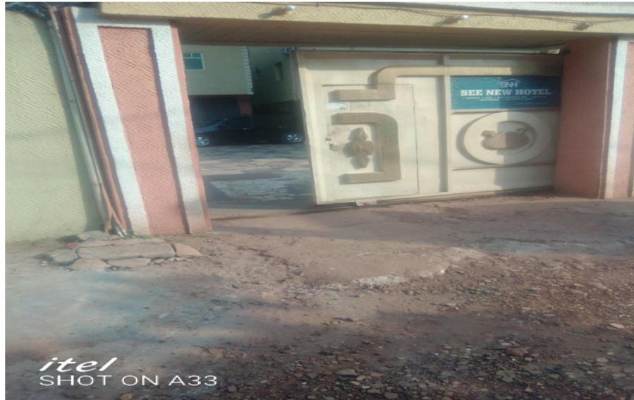
Figure 5.1 shows an entrance of an existing hotel in Nsukka Source: (Filed Survey).
