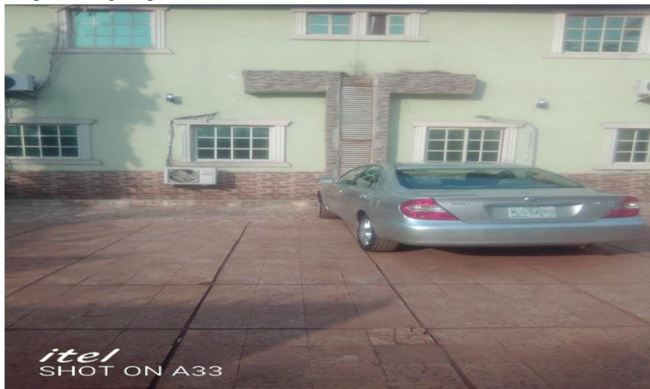
Figure 5.2 shows the state of functional obsolescence facing a hotel property in Nsukka Source: (Filed Survey).
