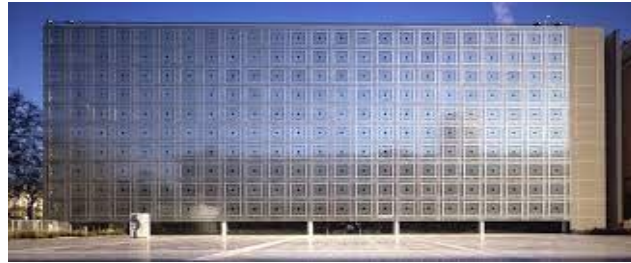
Figure 14. Southern elevation of the Arab World Institute. The developed Mashrabiyya covers the whole façade surface
