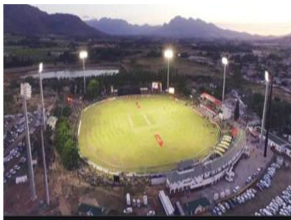
Figure 1: monopile flood light in cricket stadium.
