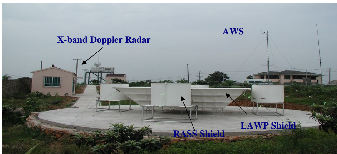
Fig.1 Wind profiler Antenna assembly
