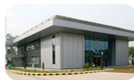
Eco Commercial Building (ECB) Bayer Material Science, Greater Noida, UP
