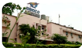
GRIDCO, Bhubaneswar, Odisha
