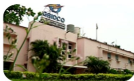
GRIDCO, Bhubaneswar, Odisha
