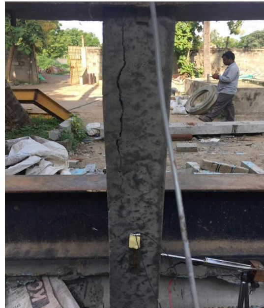
Fig.4: Steel Jacketing Setup
