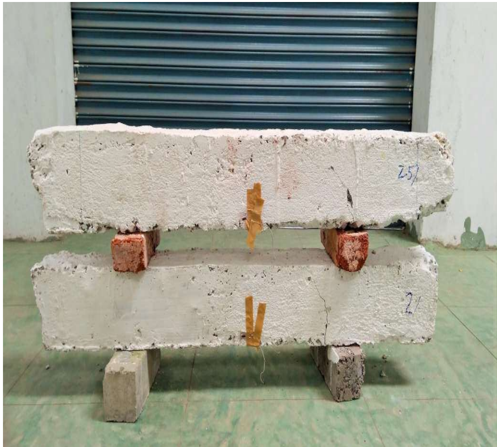
Fig 17– Crack pattern of NVC beams with 2% and 2.5 % of glass fibres
