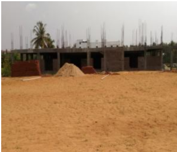
Fig 2.3 Building Front view
