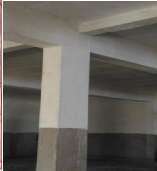
Fig 2.2 Existing structure Beam-Column joint
