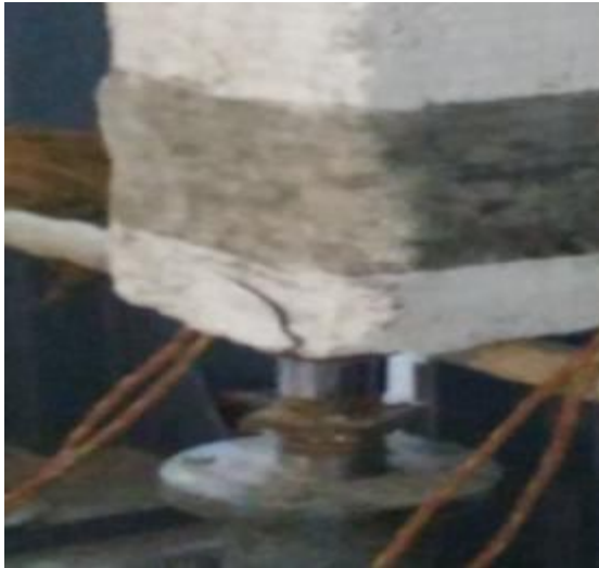
Fig 4.1.1 Cracks In Specimen B
