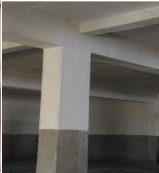
Fig 2.2 Existing structure Beam-Column joint
