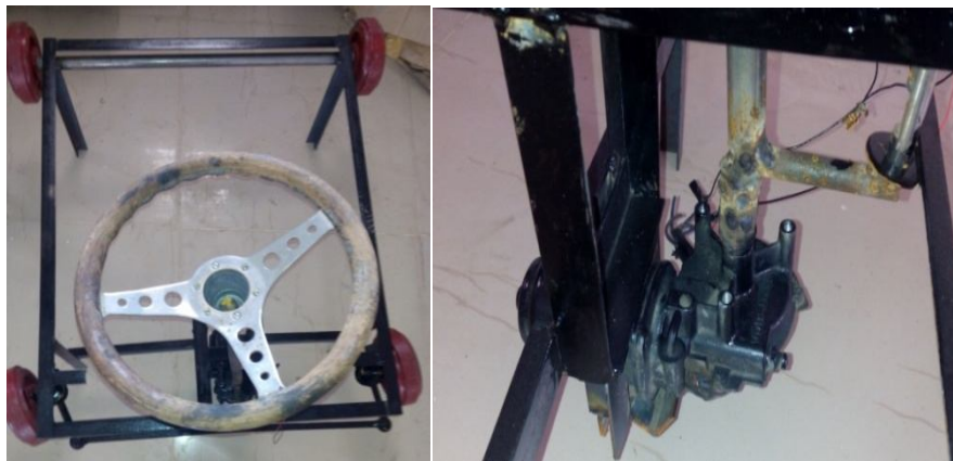
Fabrication of electrical steering mechanism
